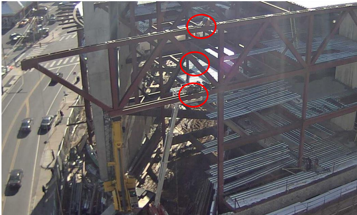
Figure 11: Full Penetration Welds Required (represented by red circles) (Picture Courtesy of Multivista.)
